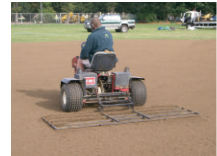
4. Grading to level
